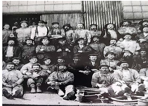
Fast Plant Dock Workers, M.A. Hanna Dock, Ashtabula
